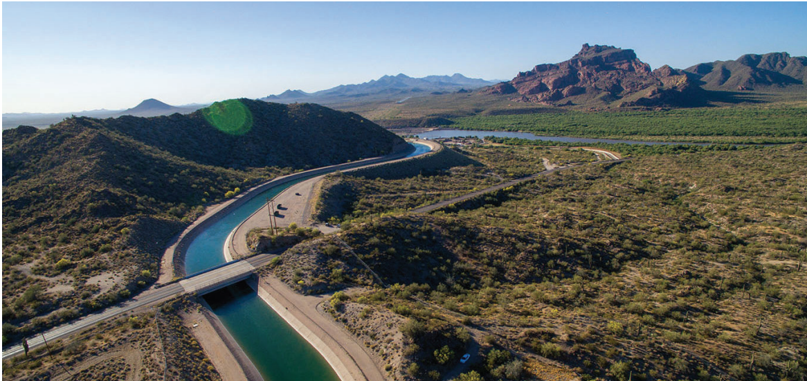
Photo: Arizona Central Project
